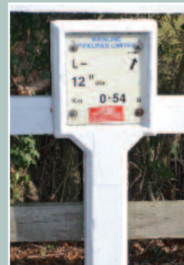
Mainline marker post
